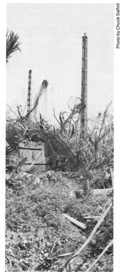
The remains of Wings of Asia . . . heavy aviary netting was torn and wadded up like thin gauze, clumps are left hanging from cables supported by these towers. Instruments on site recorded winds at 165 m.p.h. with gusts to 200 m.p.h!
