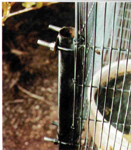
Ordinary U-bolts are used to secure the legs to the cages.
