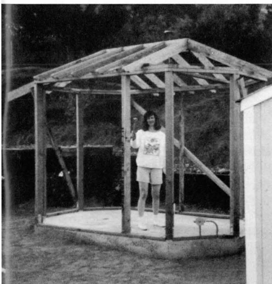
Once the concrete slab is ready, the framing goes up and the structure begins to look like an aviary. Note the electrical fixtures.
