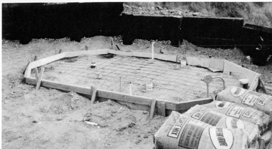
Before the foundation was poured, all the plumbing and wiring had to be figured out and installed in the correct places to be available when the concrete hardened.
