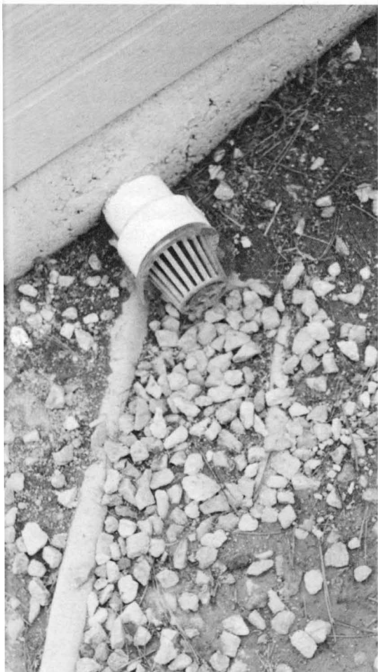
The floor wash drain system has a screening cap to filter out all seed and debris. Only clear water drains into the gravel.
