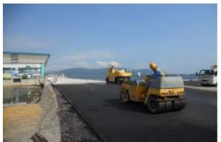
Figure 2 - Elevating and resurfacing port areas in Japan
