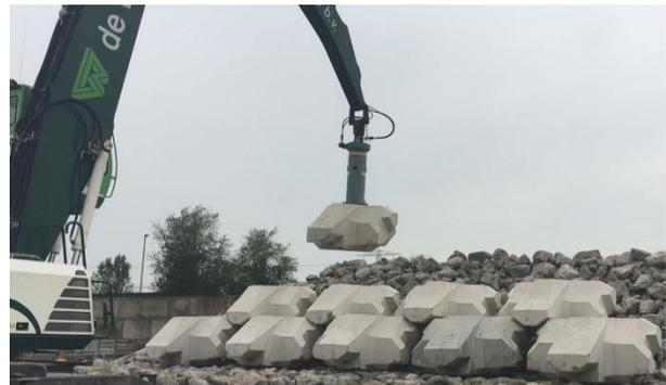
Figure 4: Placement of 6.5ton XblocPlus
