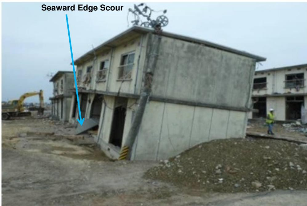
Figure 3. Damaged apartment complex at Yuriage, Natori City, Miyagi prefecture.
