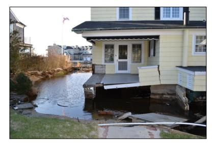
Figure 8: Foundation failure of a house on the bayside of Mantoloking due to severe scour.
