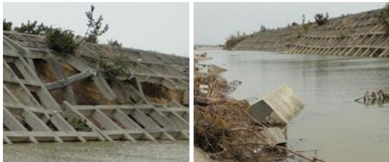
Figure 1. Coastal dikes broken by the 2011 tsunami on Yamamoto Coast, Miyagi, Japan.
