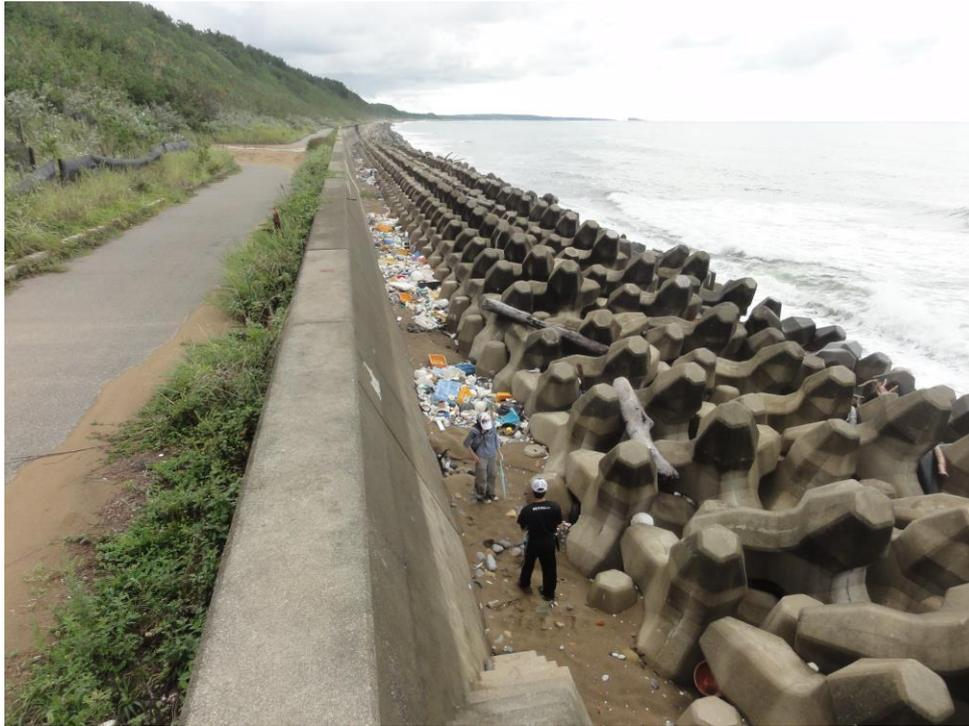
Figure 2. Eroding coast in front of the old dune on the south of the Daishoji River mouth. Seawalls are installed to decelerate erosion.
