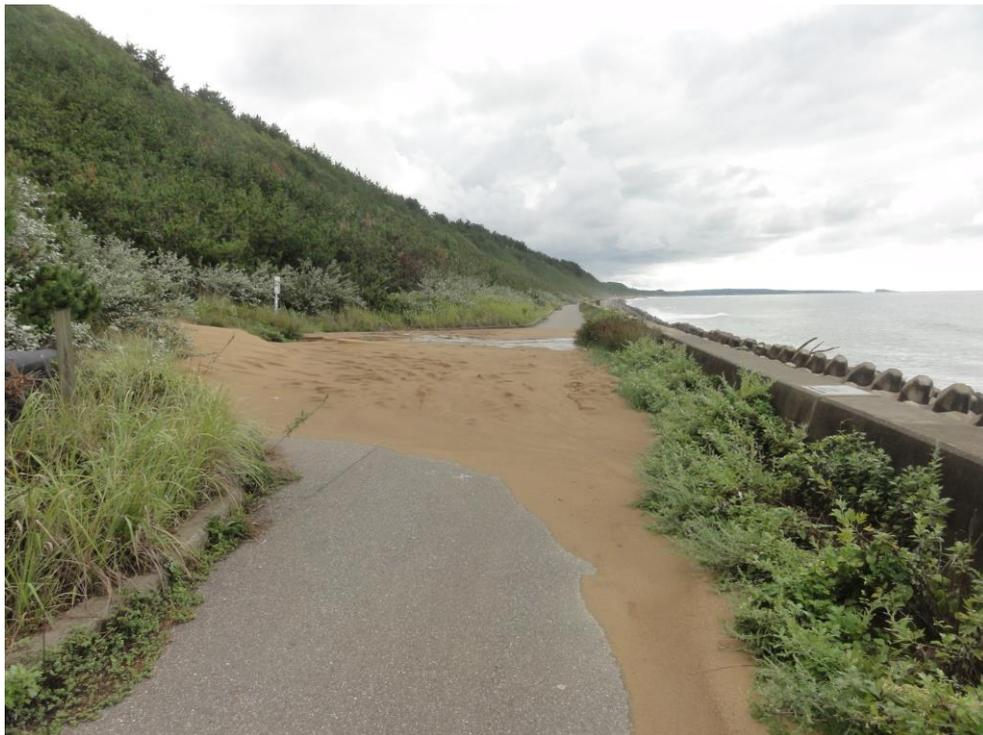
(b) Land slide sand piled up on the top of seawall
