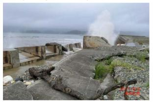
Figure 1 Collapsed seawalls due to tsunami
