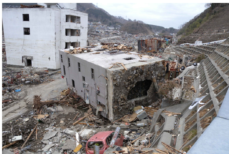
Figure 2. A 4-story RC building (7.0 m wide, 5.3 m deep and 13.3 m high) swept away about 70 m together with foundation piles of the friction type by the 2011 Tohoku Earthquake Tsunami (Onagawa in Miyagi pref.).
