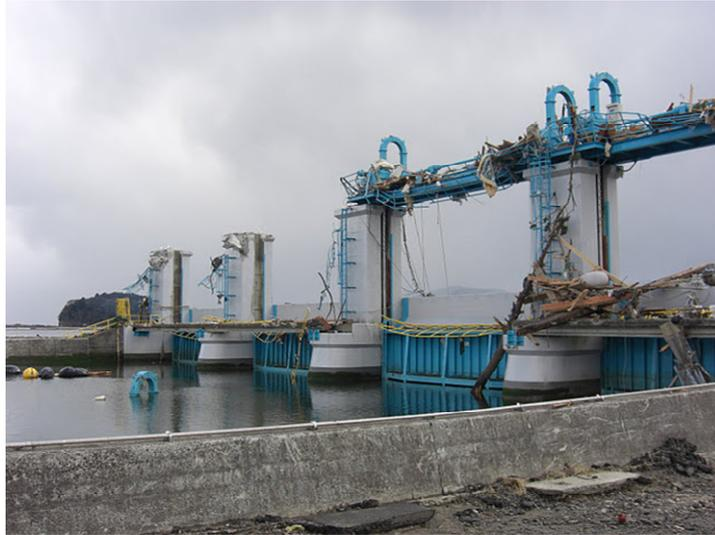
**Figure 2: Damaged floodgate at Minamisanriku**
