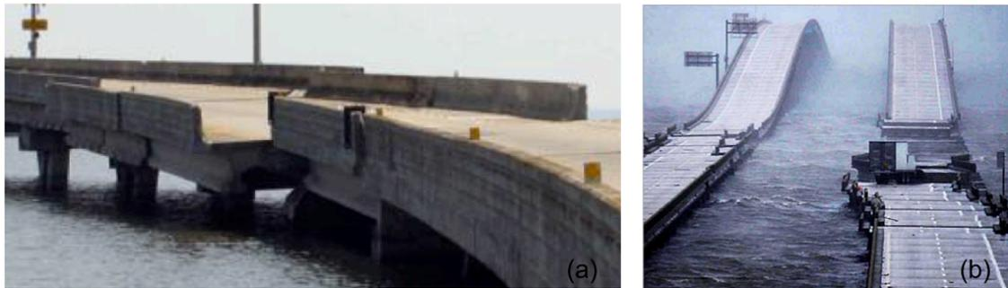
Figure 1. Pictures of damages on highway bridges after Hurricanes Katrina (a) and Ivan (b) (from Douglass et al. 2006).
