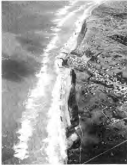
Detached breakwaters, beach nourishment and revetment
