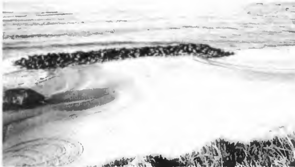
Rubble-mound breakwater
