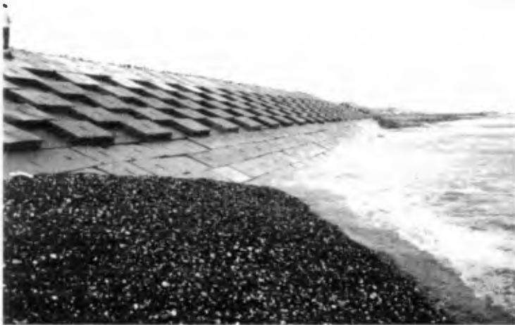
Placed concrete block revetment
