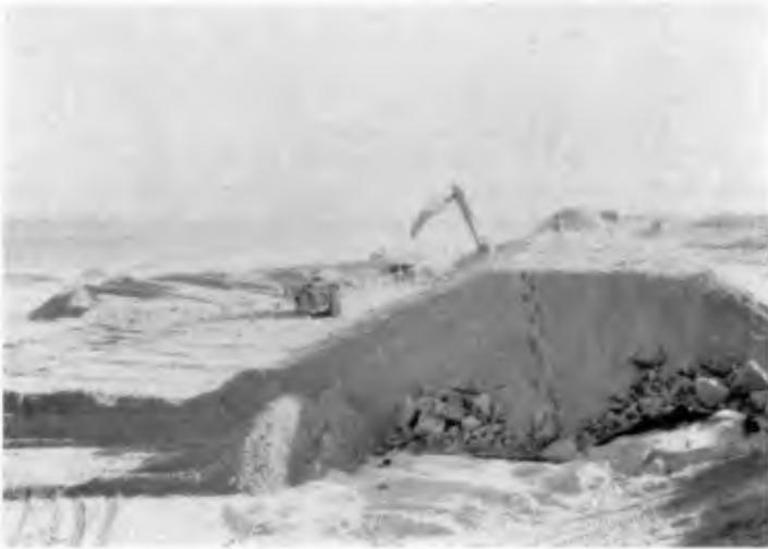
**Figure 8** Photograph of dune with buried seawall/revetment under construction
