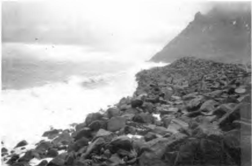
Figure 9. The Bolungarvik breakwater in 1996 after having experienced the design storm lasting for at least two days in January 1995.
