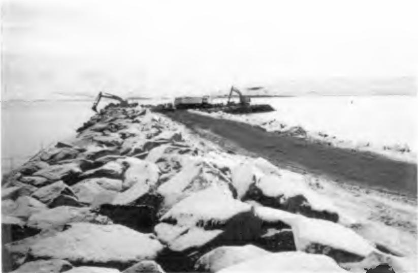
Figure 5. From the construction of the Dalvik breakwater during the winter 1994-95.
