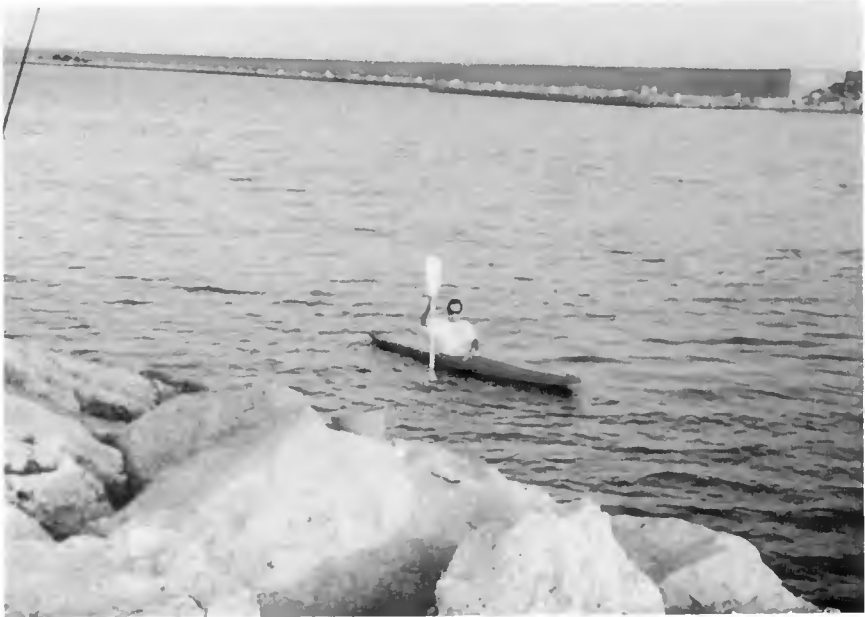
Fig.3.- Siltation at the Marina Entrance Channel.
