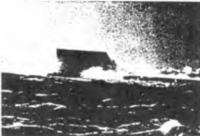
Photo 1 Wave Action on Wave Power Extracting Caisson
