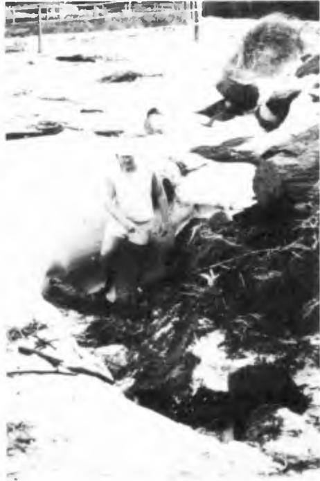
Figure 11: Scour hole formed on the beach next to the southern breakwater on 22-6-89
