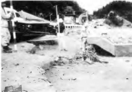
Photo. -2 Destroyed seawall and road due to storm surges (Sosu coast, Typhoon T8613)
