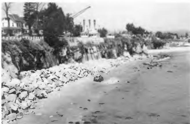
**Figure 6 - Seawall during Construction (April 1962)**
