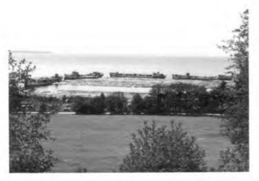
Fig. 5. The floating breakwater at Powell River, comprised of ship hulls.
