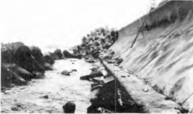
Photo 8. First, mound of armour units were removed.
