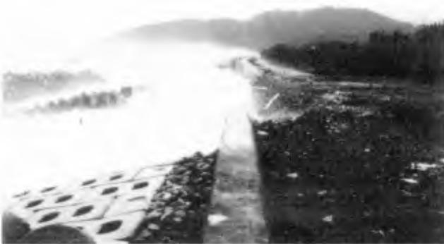
Photo 12. Heavy waves overtopped the crown of the experimental seawall, on the 20th December 1986.
