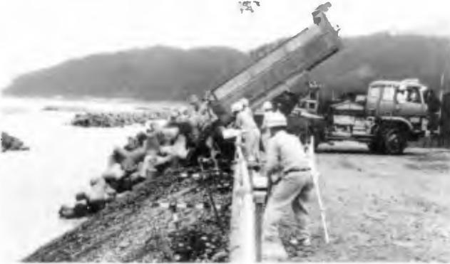
Photo 9. Filling of sand and gravel, which were diverted from the dredging of Miyazaki fishing port, located 4 km away from the site ( cf. Fig.7 ).
