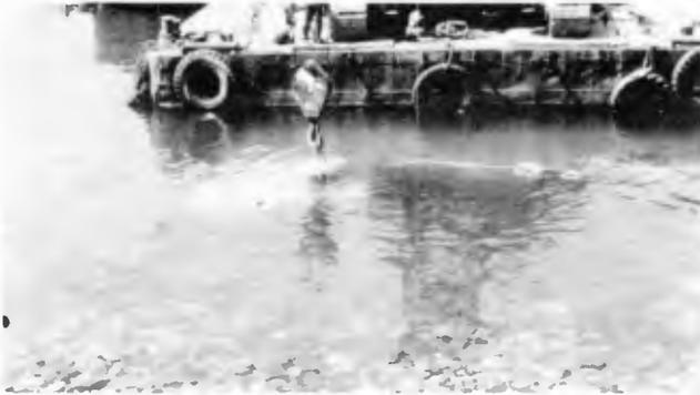
Photo 10. Setting the Lotus-Uniblock on the rubble stone. The lowest block were set at -3.3 m water depth.
