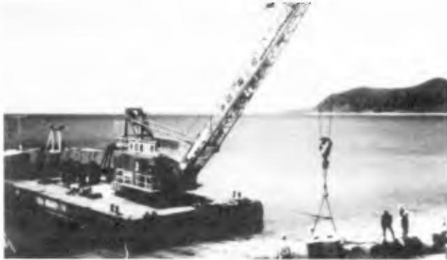
Photo 5. The experimental seawall under construction.
