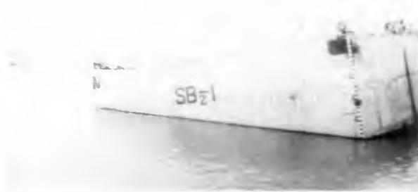
Figure 6. Caisson slides toward water under process of Slide-to-Float method
