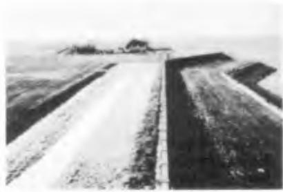
Fig. 4 Eastern Scheldt dike (with return wall)
