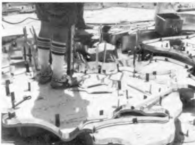
clamped to the angles, surveyors confirming the accuracy of the clamping and technicians with a portable spot welder fastening the ribbons permanently in place.
