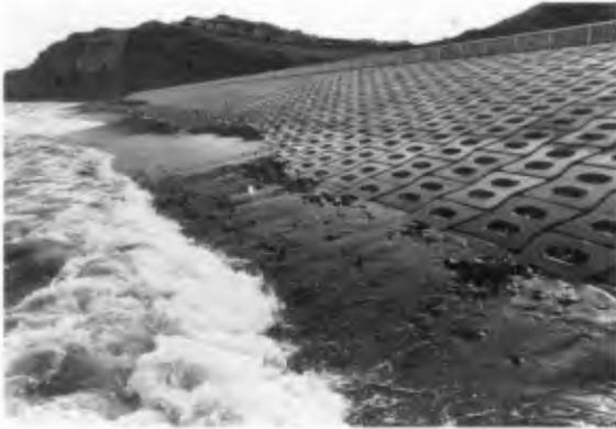
Photo.8 Gravel are left on the toe of the seawall
