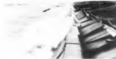
Photo.1 Backfill sand is drawn out
