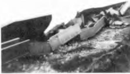
Photo.2 Vertical type seawalls collapsed
