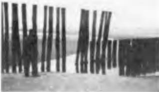
FIG.18 Pulled piles
