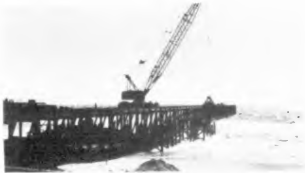
Figure 7 SURF ZONE TRESTLE
