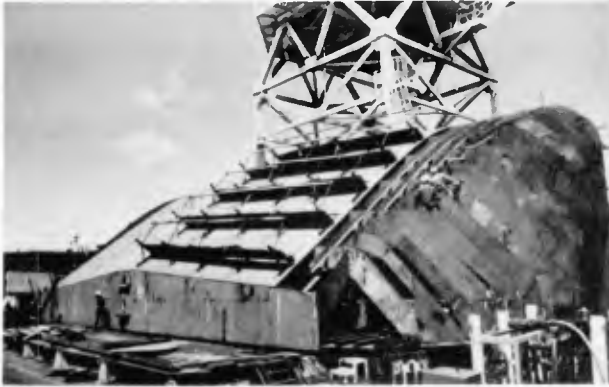
Figure 14 BARGE DURING CONSTRUCTION
