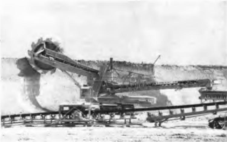
Plate 2. Bucketwheel Excavator.
