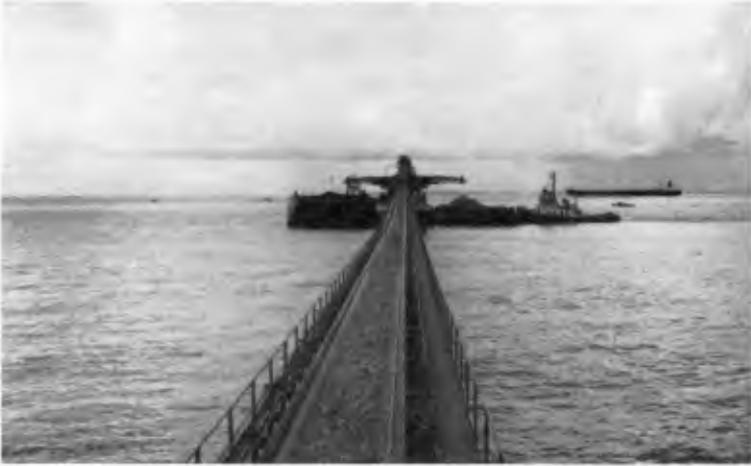
Plate 3. Loading of fill material from the belt conveyor onto barges.
