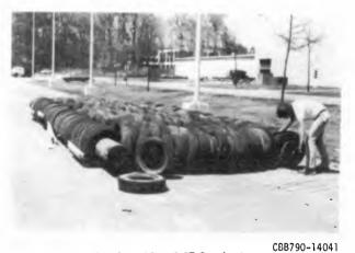
Plate 2. Assembly of PT-Breakwater.
