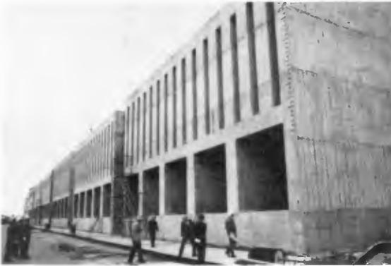
Fig. 16.- Completed Caisson for Seawall
