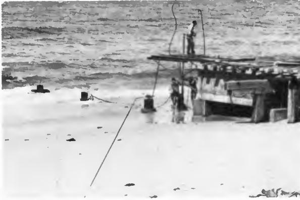
FIGURE 5 JACKETS BEING JETTED IN AROUND PILES
