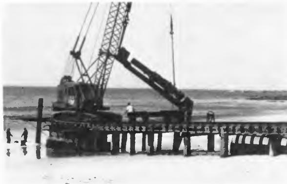
FIGURE 4 PILE DRIVER BEING LIFTED INTO POSITION
