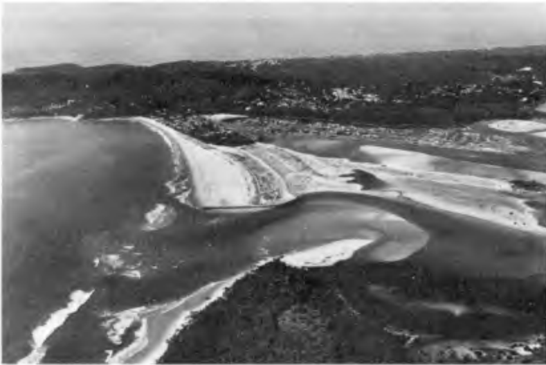
PHOTOGRAPH 1 - The completed scheme (August 1979)
