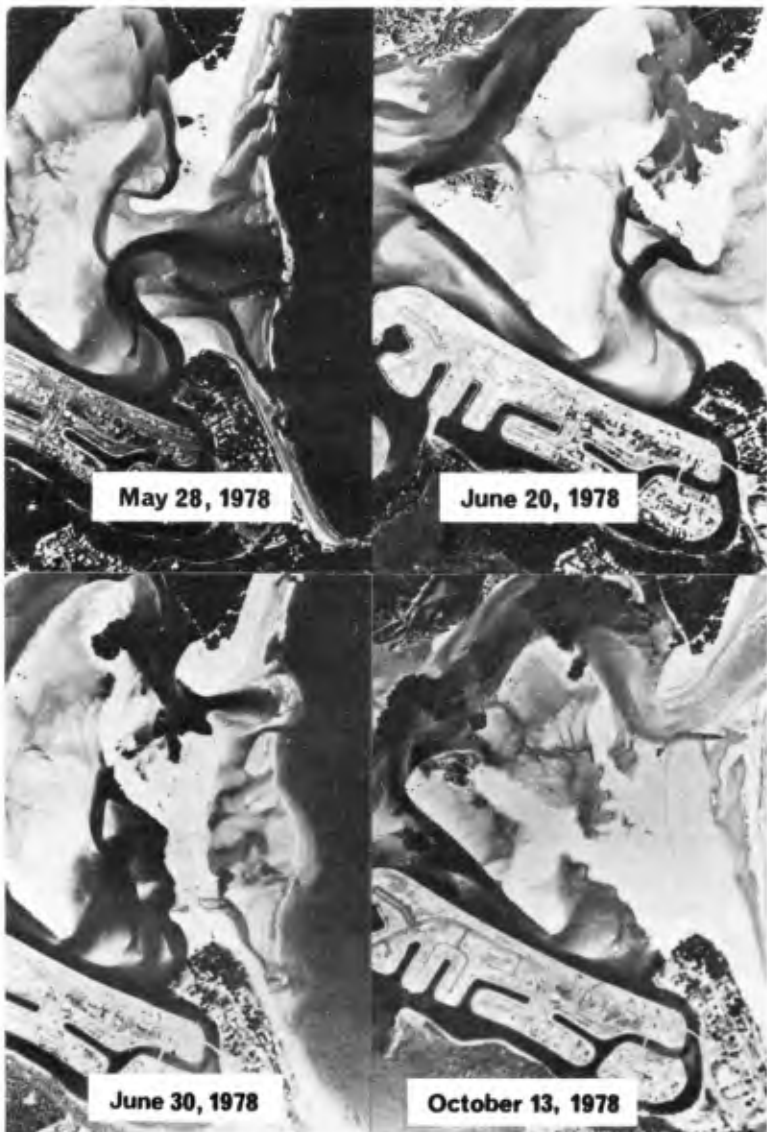
FIGURE 5 - Photographs showing progress of the works
