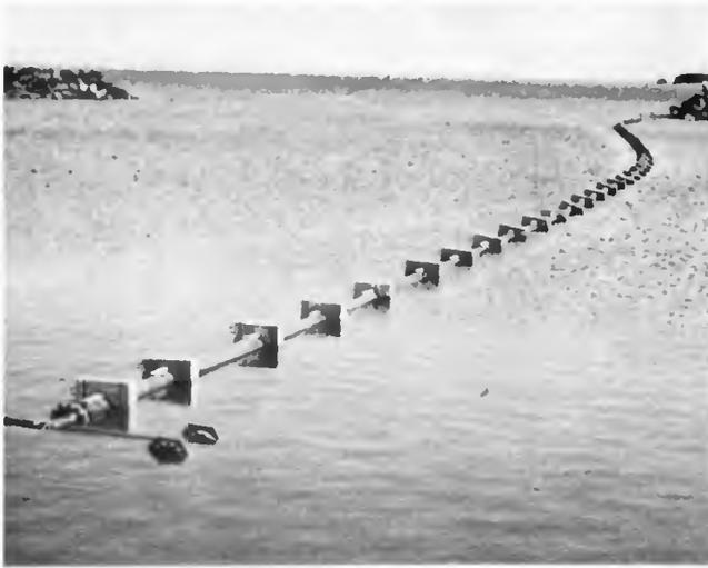
**Figure 23. Launching Outfall by String Float Method.**
