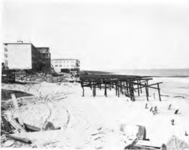
Figure 2.—Boardwalk at Rehoboth Beach, Del., destroyed by the March 1962 storm.
