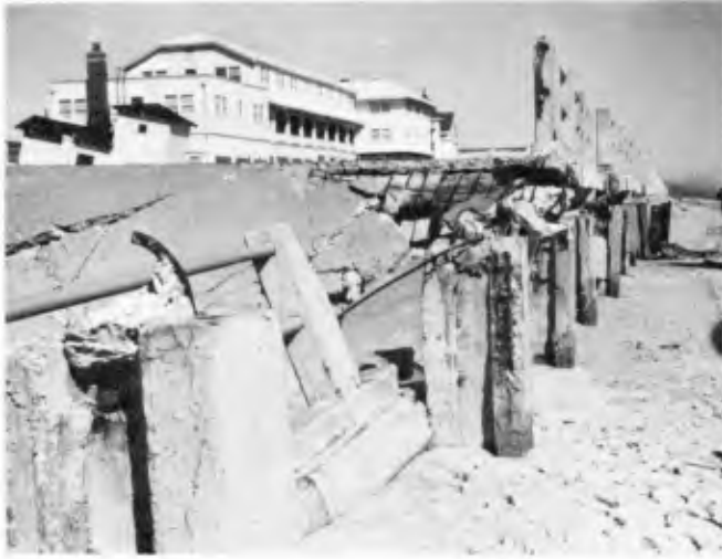
Figure 1.—Damage at Virginia Beach, Va., caused by the Severe March 1962 storm.
