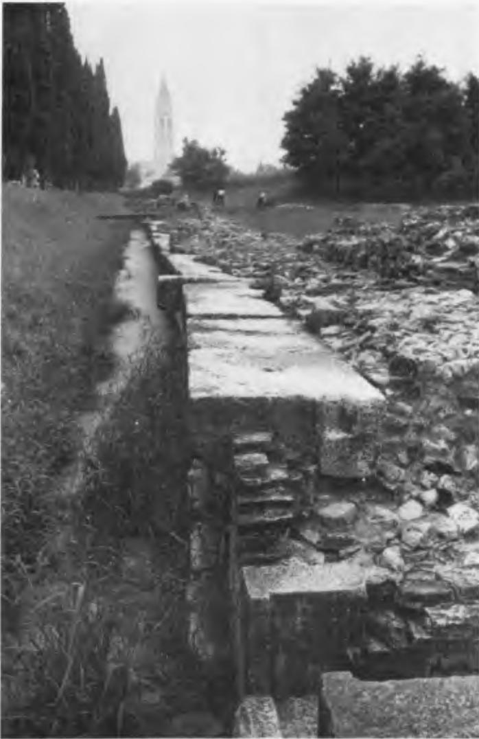
Figure 7. Stone quay in river port of Aquileia, Italy (circa 180 B.C.). Quay had landing stages at two levels (for varying river levels?). Note protruding mooring stones shown in Figure 8.
