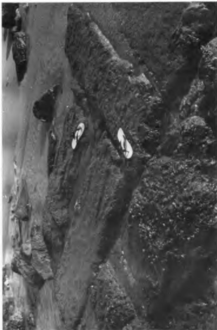
Figure 6. Phoenecian quay at Atlit showing interlocked and offset slabs where the breakwater joins the quay wall.
