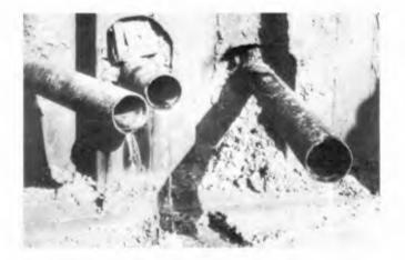
Fig.2: Auger-bored inclined drains lined with pitch fibre pipes ready for connection to the collecting toe drain.
