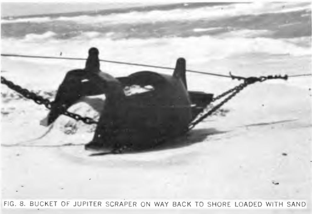
photography is also being used to observe the operation as well as the development of the borrow area after operation has been shifted to another area. The coastal protection at Jupiter Island is a combination of artificial nourishment by hydraulic dredge from the intracoastal waterway and lagoon behind the barrier, some short adjustable groins and revetments as described in ref. 8.
