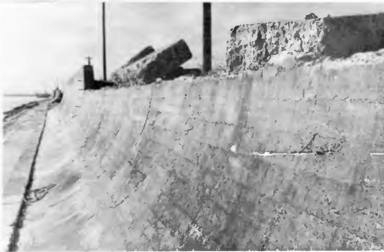
Photo.4.5 The overturning of parapet in the coastal dike at the left side of Nikko River.
