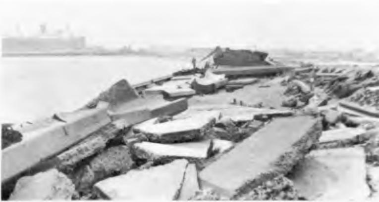
Photo.4.3 The damage of Isozu coastal dike.
