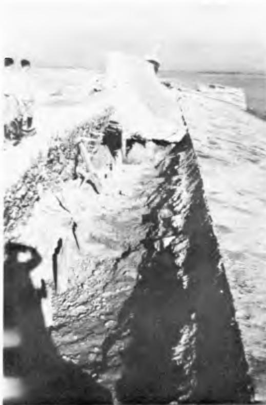
Photo.4.4 The damage of Koeishinden coastal dike at Handa.
