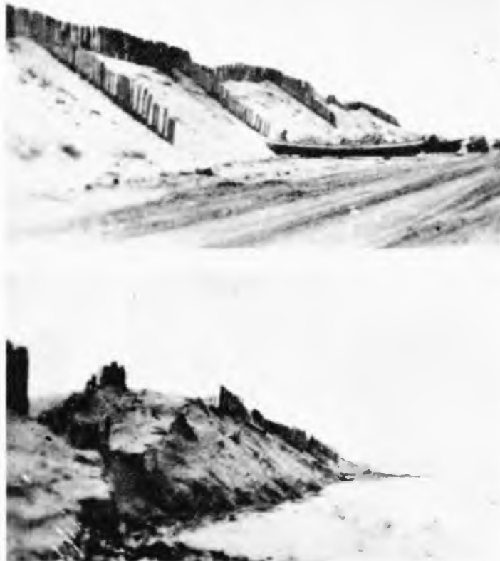
Fig. 5 - The first artificial dune near the sea, a) before the hurricane, b) during the hurricane.
