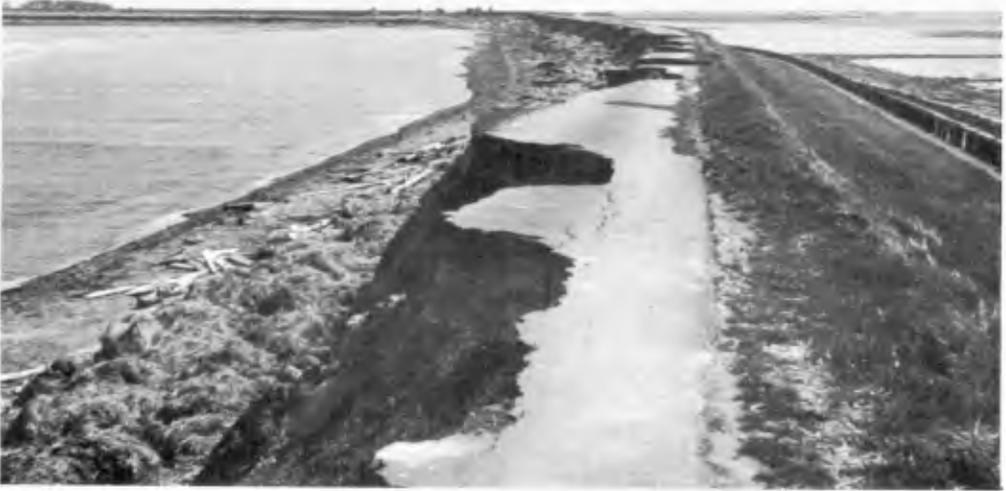
Fig. 11. A damaged dike. The sea is on the right and the land was to the left. Damage occurred at the inner side.
