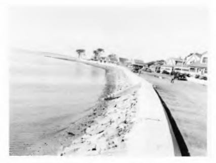
Fig. 5. "Permeable Seawall".
