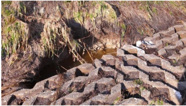
Figure 19. One of the holes undermining the maintenance road
