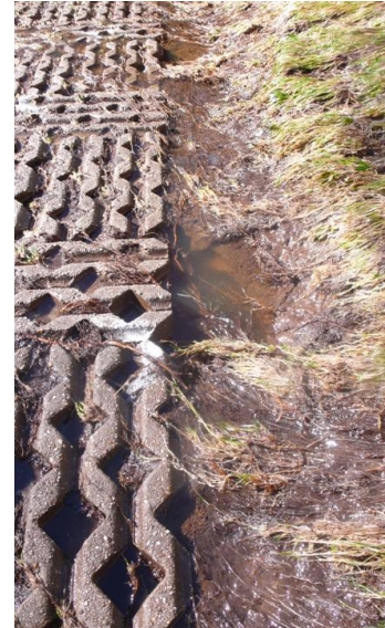
Figure 18. First damage at upper edge of maintenance road
