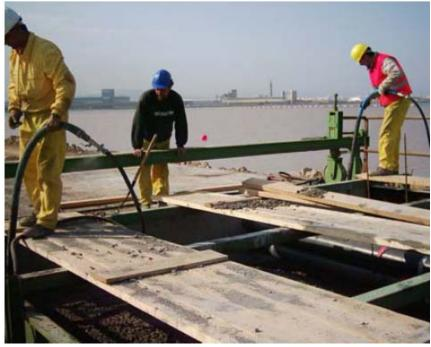
Figure 11.- Superstructure execution over quay wall caisson
