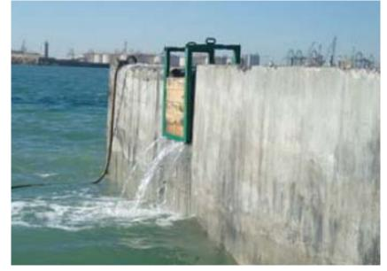
Figure 10.- Cap used for closing external windows in caisson.
