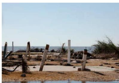
Figure 1 - House pushed over by flood loads during Hurricane Ike. The failure occurred at the connection level between the floor beam and the piles (FEMA 2009).
