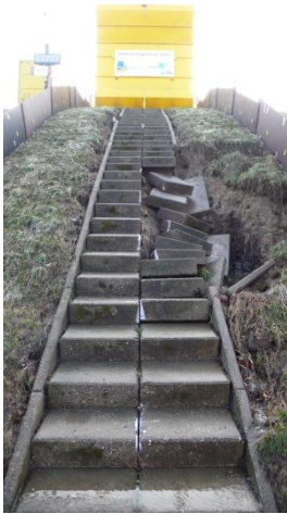
Figure 9. Failure of stairs, section 2
