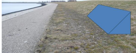
Figure 4 Excavated part of the seaward slope (for maintenance block revetment lower end of slope)
