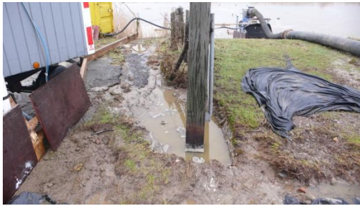
Figure 14. Scour around pole 0.2 m, section 3
