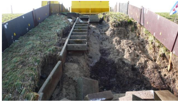
Figure 10. Destruction of stairs
