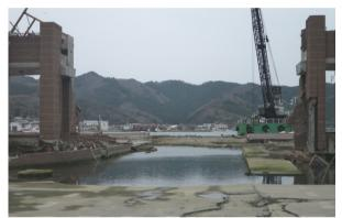
Photo 10. Local scouring between two wings of Marinpal Onagawa (The photo was taken on April 26, 2011.).
