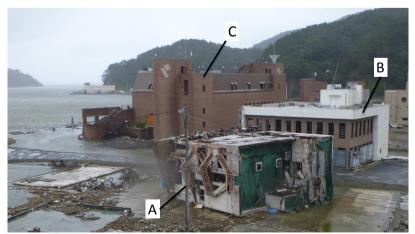
Photo 8. Example of damaged reinforced concrete buildings in Onagawa Town, where Building A is toppled down not behind Building C, i.e., the north wing of Marinpal Onagawa (The photo was taken on September 21, 2011.).
