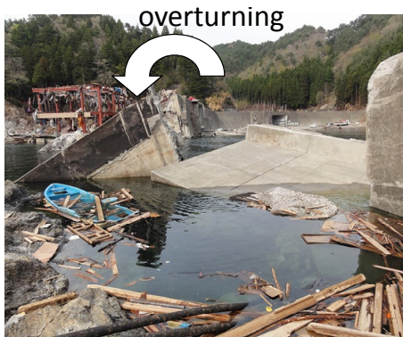
Figure 15. Overturning of seawall on Ryoishi Coast, Iwate Prefecture.
