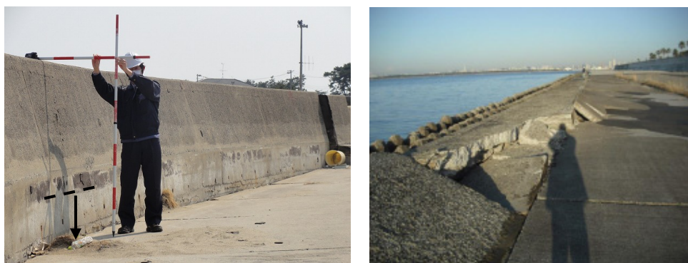
Figure 17. Examples of damage mainly caused by seismic motion (left: Yotsukura Coast, Fukushima Prefecture; right: Ichikawa Coast, Chiba Prefecture).
