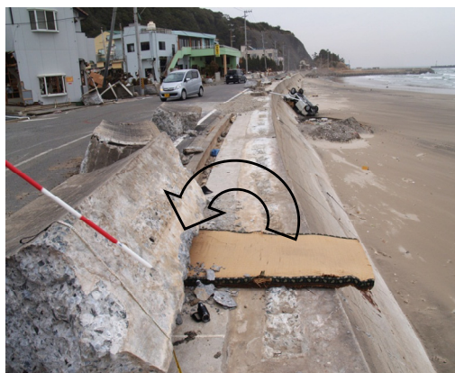
Figure 11. Parapet failure on Toyoma Coast, Fukushima Prefecture.
