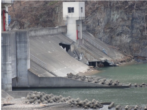
Figure 13. Failure of seaward armor on Mizuumi Coast, Iwate Prefecture.
