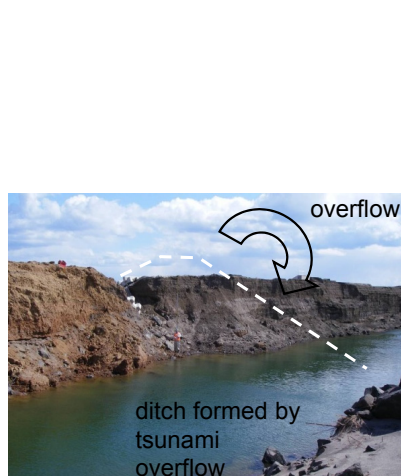
Figure 3. Ditch formed by tsunami overflow (Kabasaki Coast, Miyagi Prefecture).
